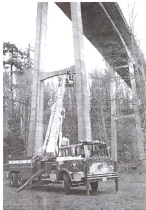
Saltwater Park Bridge is inspected following the earthquake.
